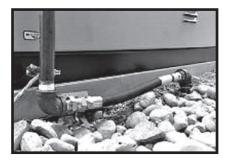
When connecting the gas line to the generator, use a short section of UL Listed or AGAapproved flexible fuel line in accordance with local regulations. The purpose of the flexible fuel line is to ensure that vibration from the generator does not cause a gas leak at one of the connection points, so it's important that the line be installed with as few bends as possible.
